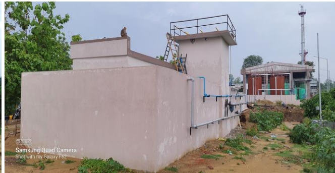
Pics.: 60 KLD ETP Based on UASBR Technology (Parag Dairy)
