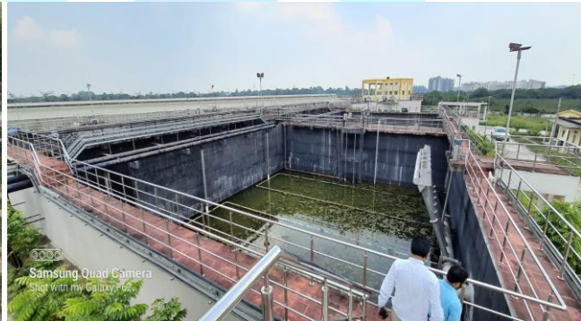
Pics.: 600 KLD STP (SBR Technology Based)
