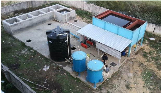
Pics.: 250 KLD STP (MBBR Technology Based)
