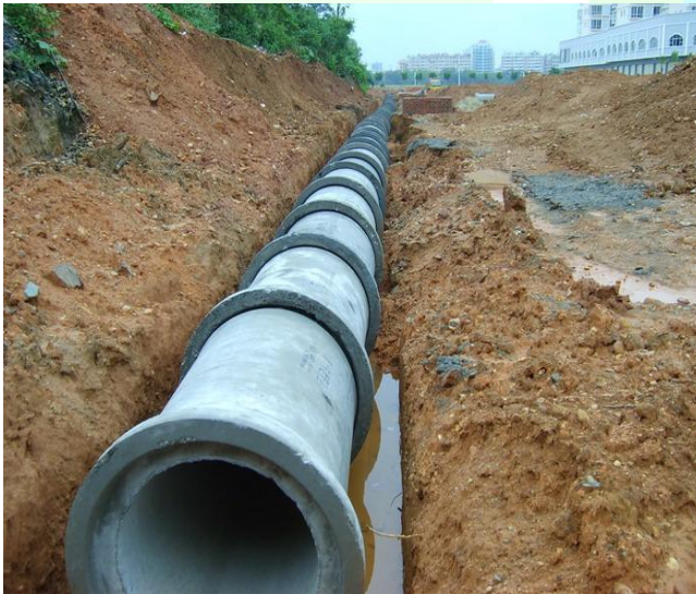
Pics.: Sewerage Line – Connection
