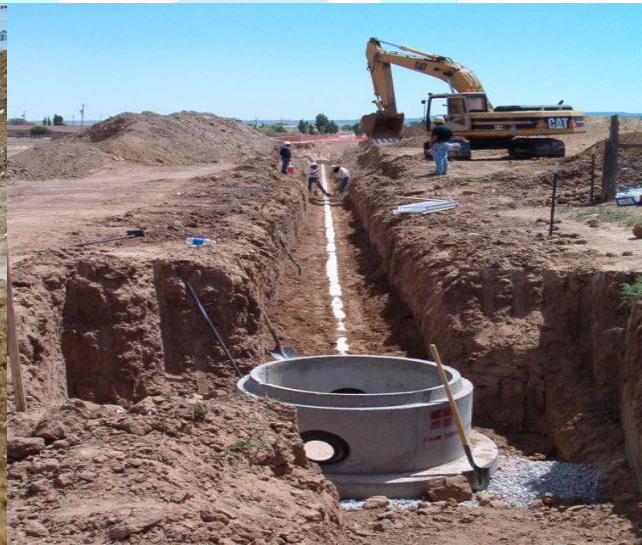
Pics.: Sewerage Line – Design & Laying
