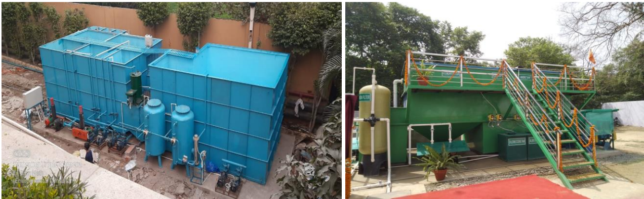
Pics.: Pre-fabricated Compact Sewage Treatment Plant
