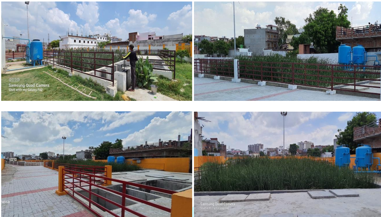
Pics.: 01 MLD & 600 KLD STP (based on Constructed Wetland Technology), Nagar Nigam
