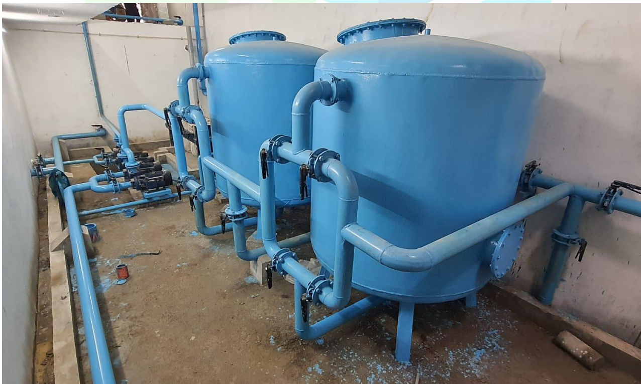
Pics.: Multi Grade Filter & Activated Carbon Filter
