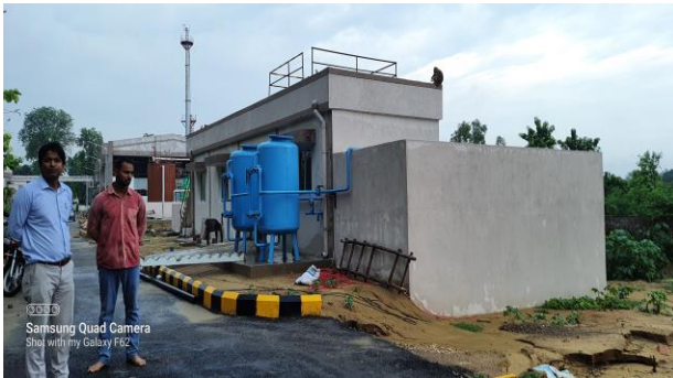
Pics.: 60 KLD ETP Based on UASBR Technology (Parag Dairy)
